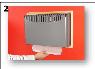
Raise the notch to release the filter and take it out from underneath. Repeat the same operation in reverse for the replacement.
