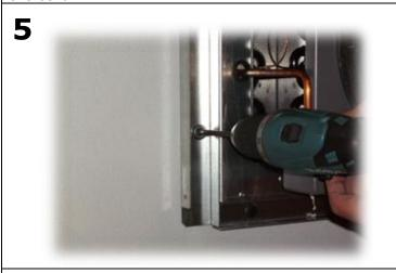
Tighten the two screw/washer units on the side
