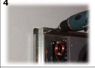
Position the air-conditioner in the frame from inside the cellar
