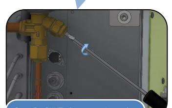
Step 3: SHUT the expansion valve fully (turn the screwdriver clockwise). Check the position of the tip of the screwdriver (to give it the right number of turns for correct expansion valve adjustment)
